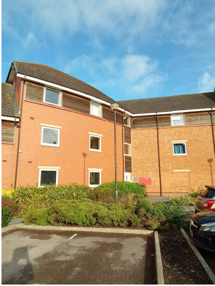
Exterior Structure (The Building)
